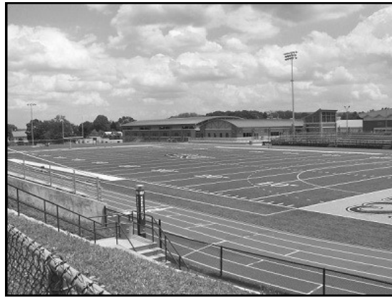
Facility Features: 2 shot put circles, 2 discus circles, and ample room for javelin training
